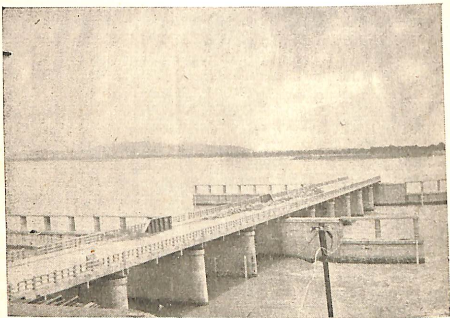
A view of Mundali weir
